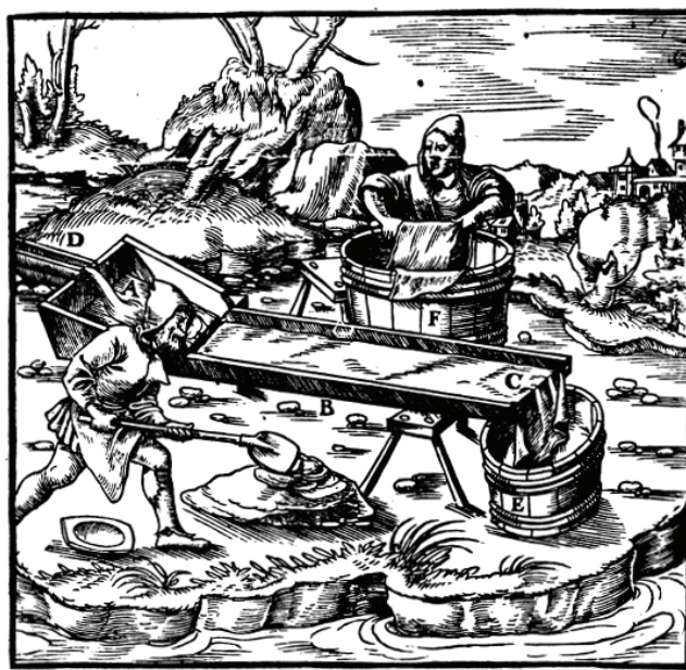
Fig. 17. Etching from De re metallica , illustrating the sluice. A: Top of the table, B: Table, C: Rag (textile), D: Pipes, E: Collection tank for rubbish, F: Tank for textile washing (After: Agricola 1530, 264).
